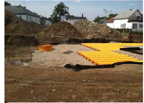
Subsurface Infiltration System
