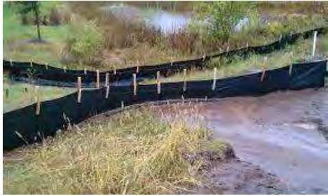
Double Row of Erosion Control Devices (Steep Inclines)
