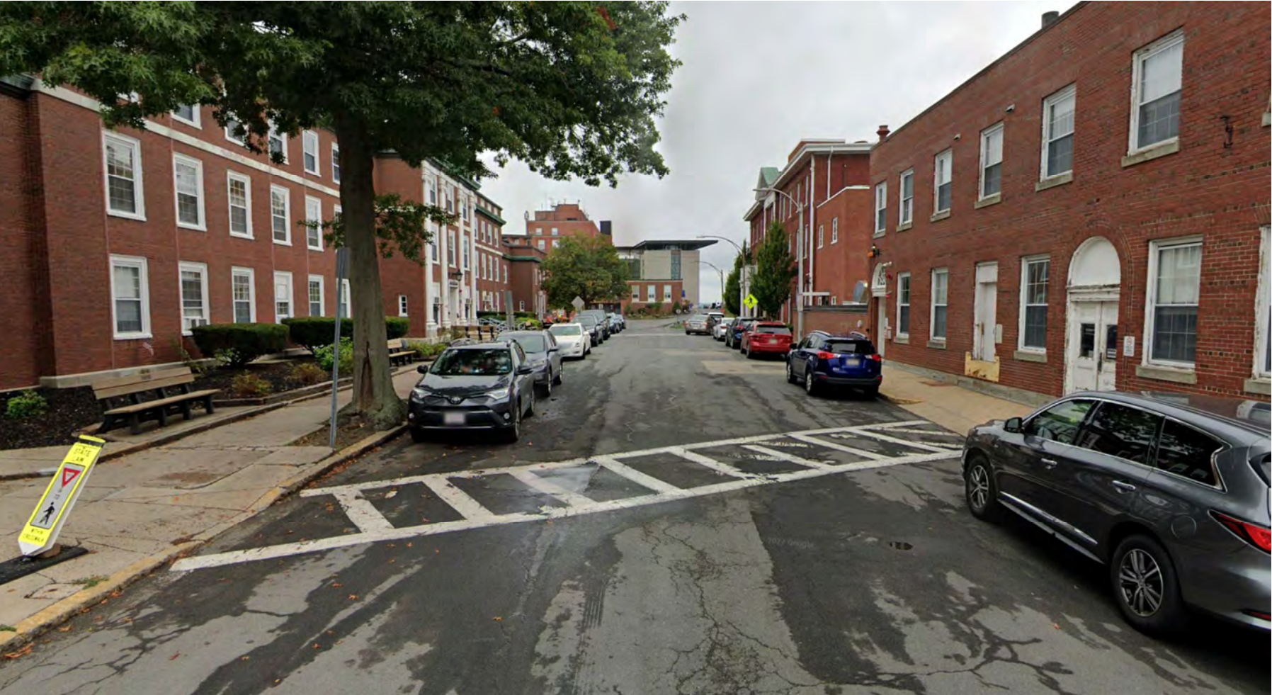
EXISTING CONDITIONS – CREST AVE.
